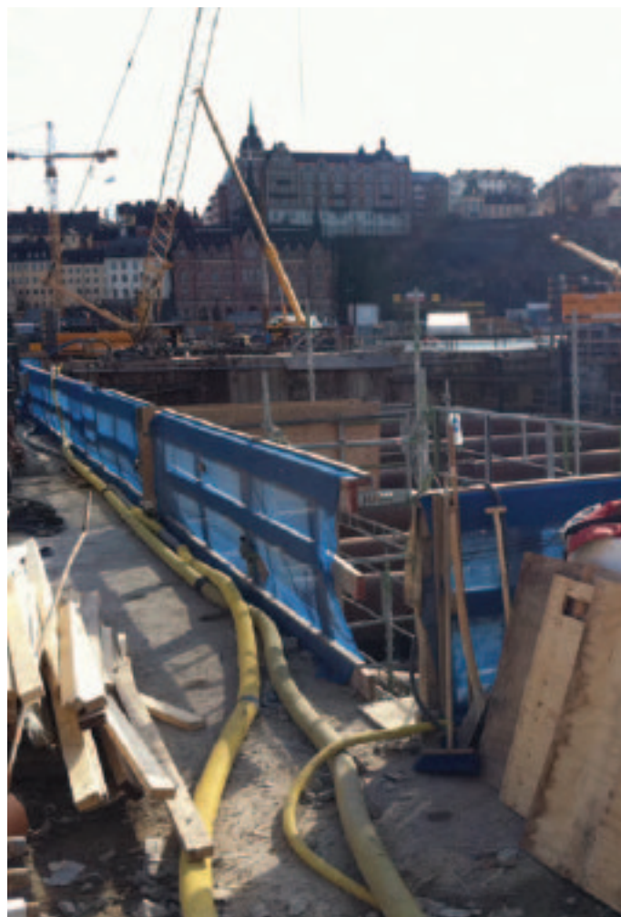
Six Tsurumi LH series high-head dewatering pumps were used in a tunnel project in Stockholm, Sweden.
