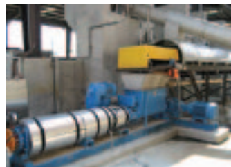
The seepex dewatered sludge pump handles up to 35 percent dry solids content. Photo by seepex.
